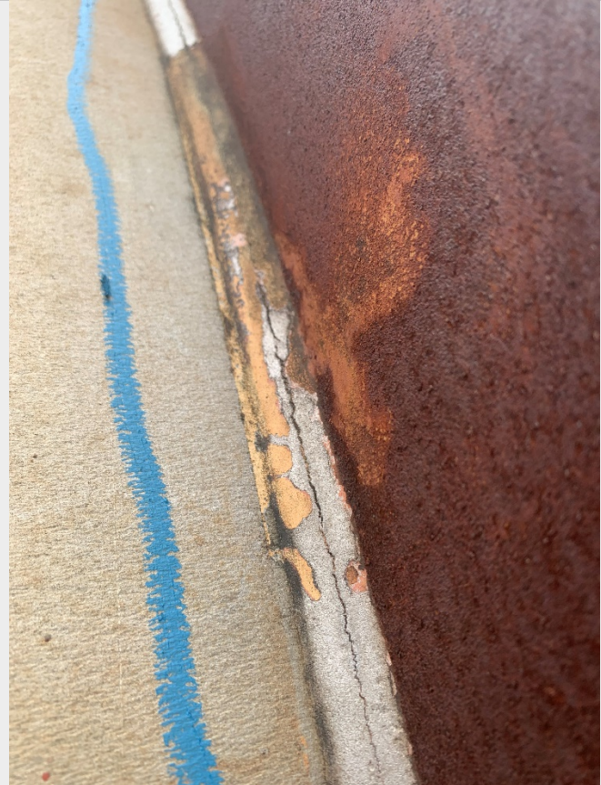
Close up view of crack like indication between the shell and stiffening ring
