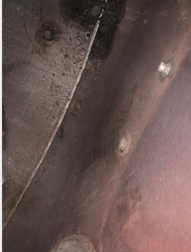
Sample view of shell to head weld
