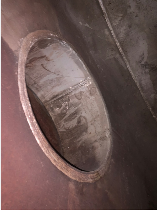
Internal view of manway (No Damage)
