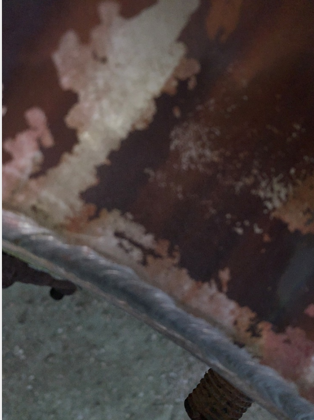
Sample of manway to shell weld condition
