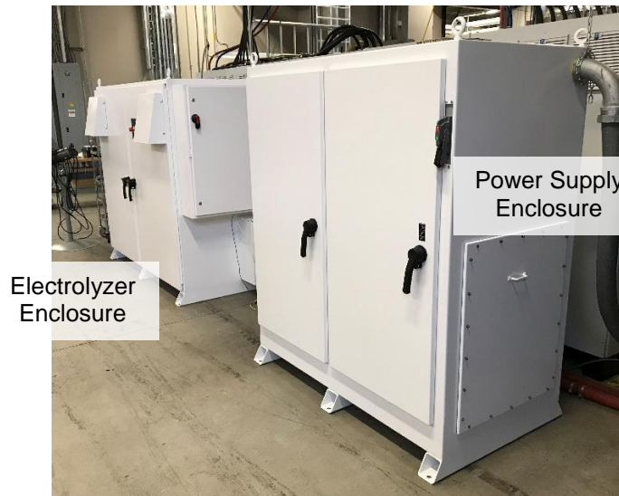
Figure 1 - C Series Hydrogen Generator
