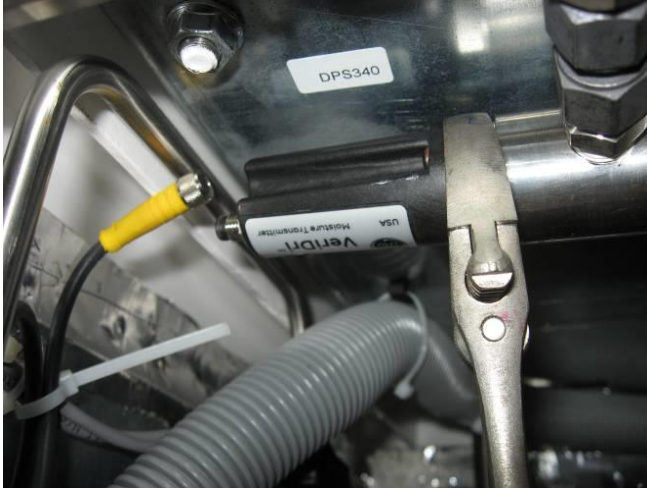
Figure 57 - Dew point sensor replacement
