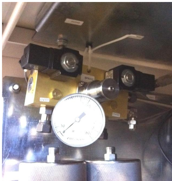
Figure 39 - Lifting the Top Manifold
