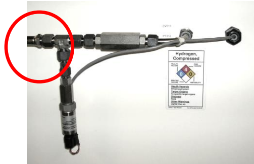
Figure 22 – H 2 Product Output Connection
