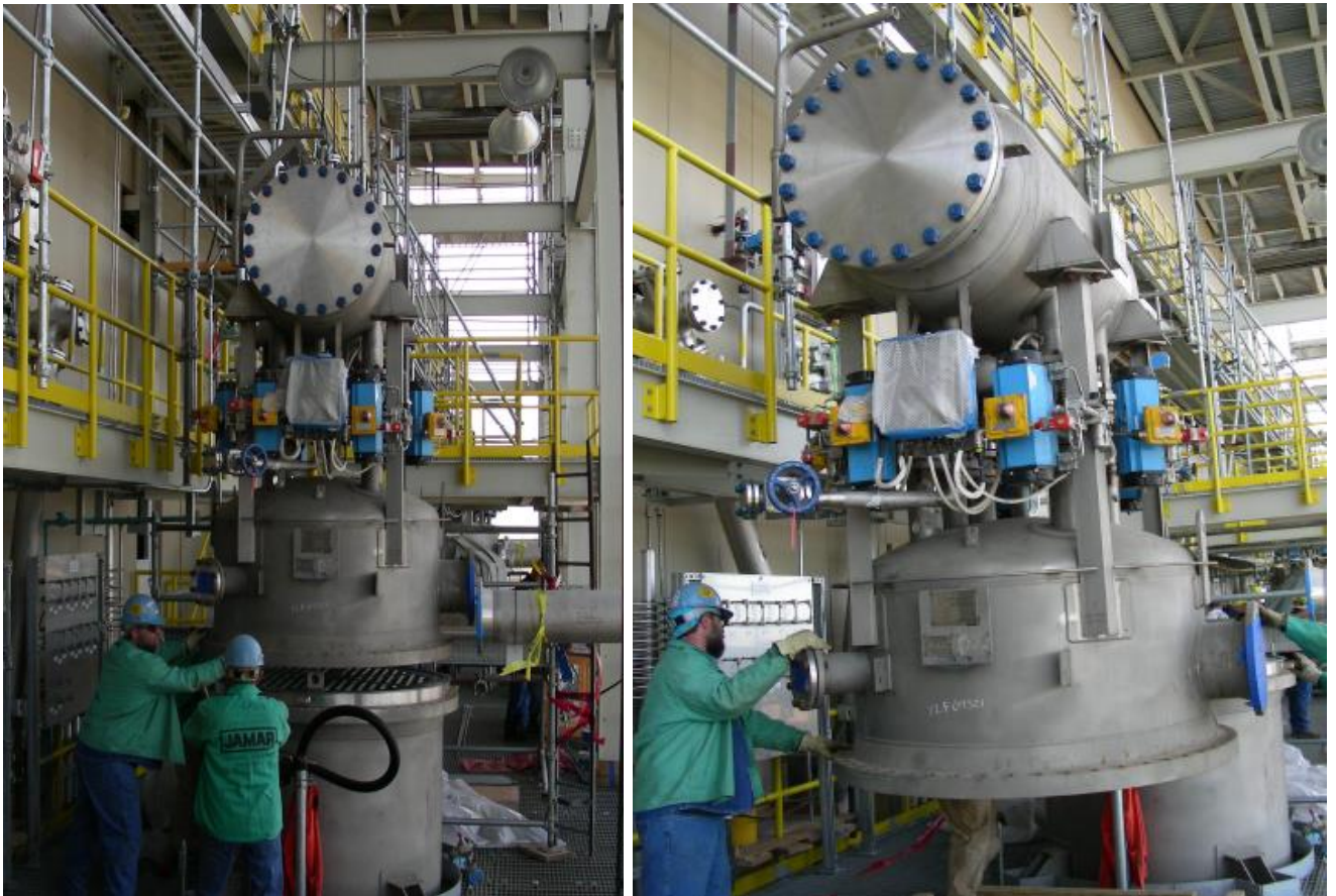
Figure No. 4.4: Typical Top Head Bonnet Removal w/ Quick Disconnect J-Box
