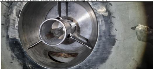
Verified shaft's limiting device is properly installed with one slot facing to nozzle N01.
