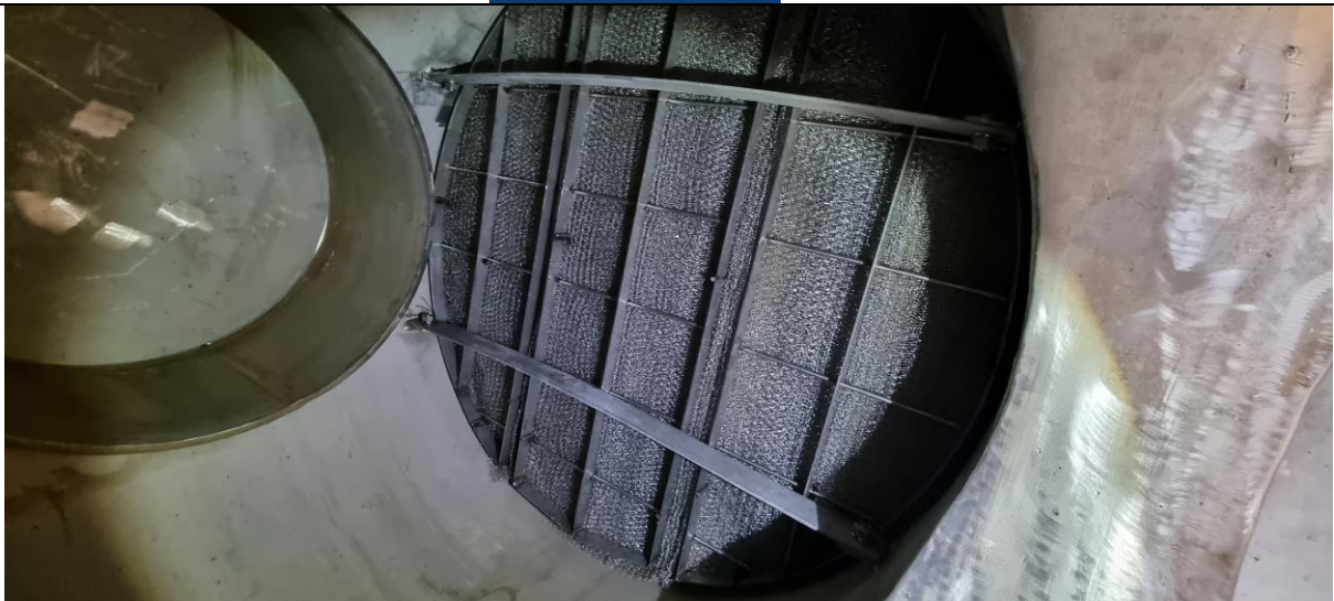
682B.2 Demister is installed.
