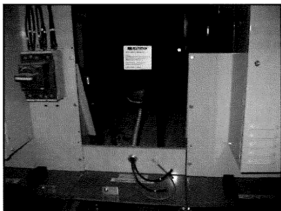
1. Remove the buss duct covers.
