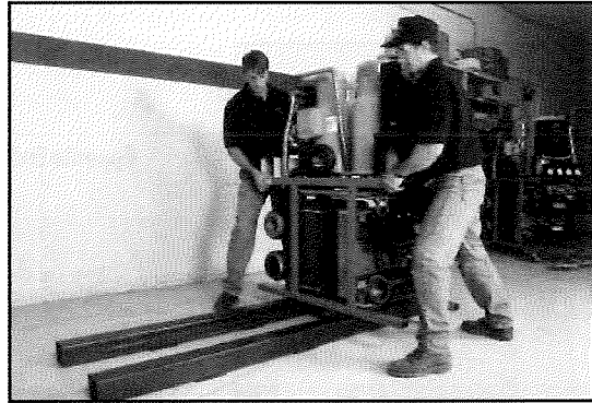
6. Slide module into position.
